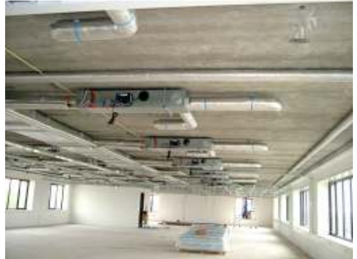
Typical lay-out Induction-VAV system
